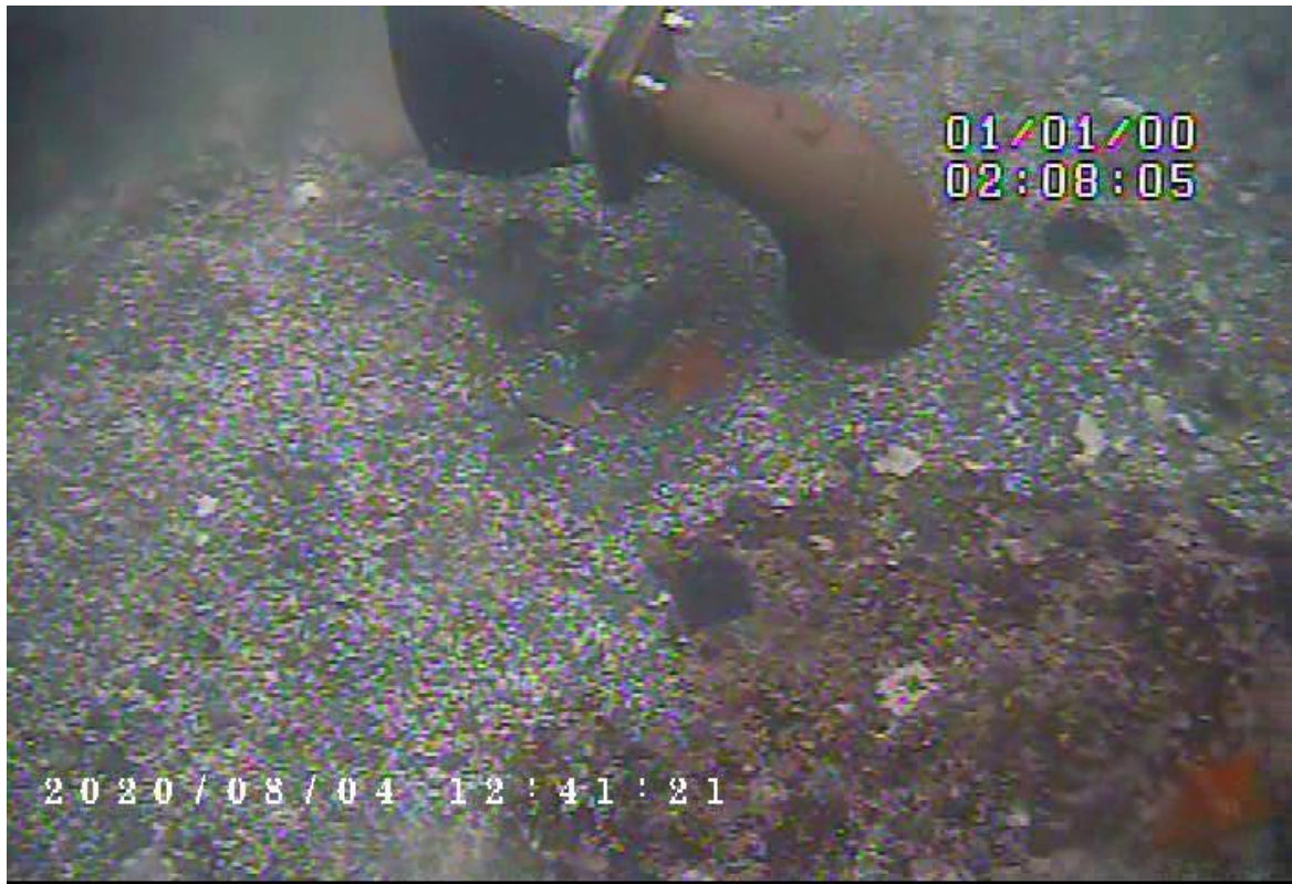
Photo 4 – Diffuser 12 showing strong flow
