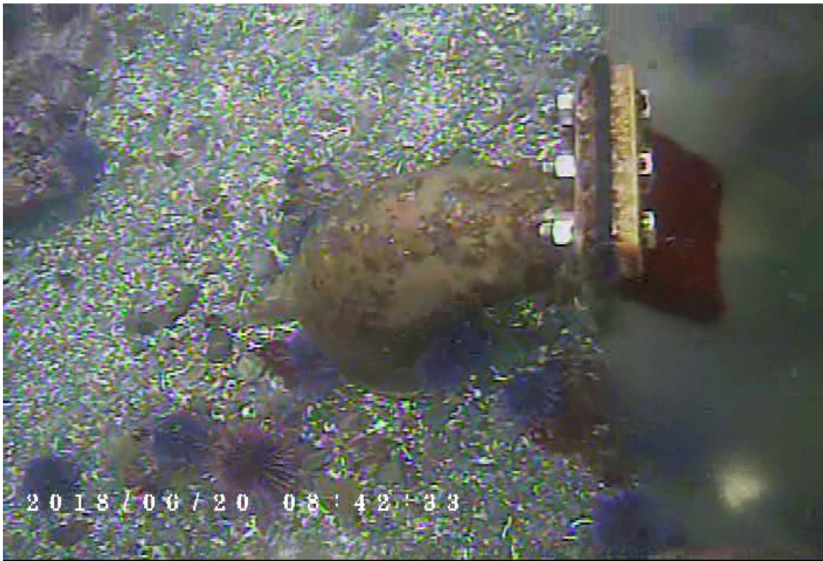
Photo 2 – Diffuser 2 showing strong flow
