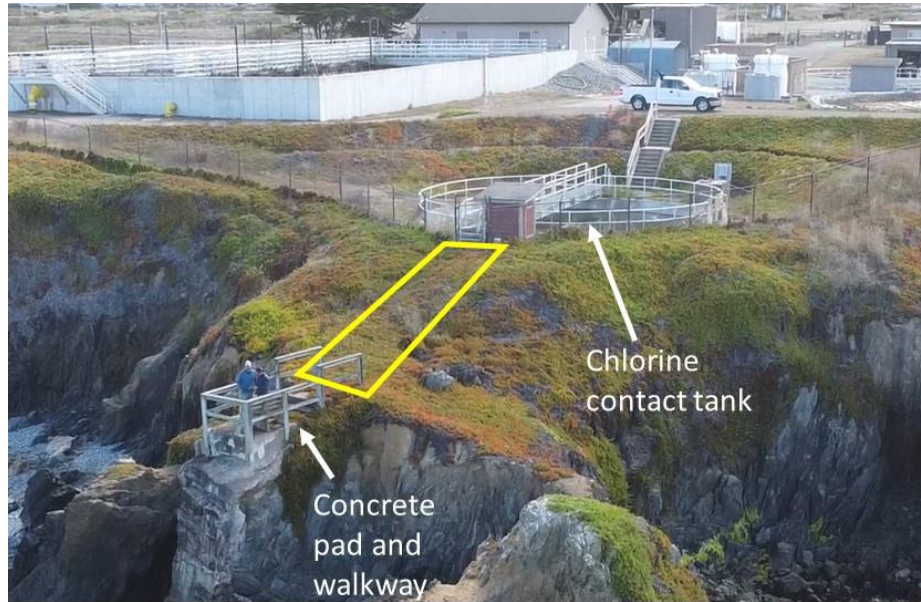
Figure 7. Vegetated area between the concrete walkway at bluff edge and the chlorine contact tank at the WWTP.
