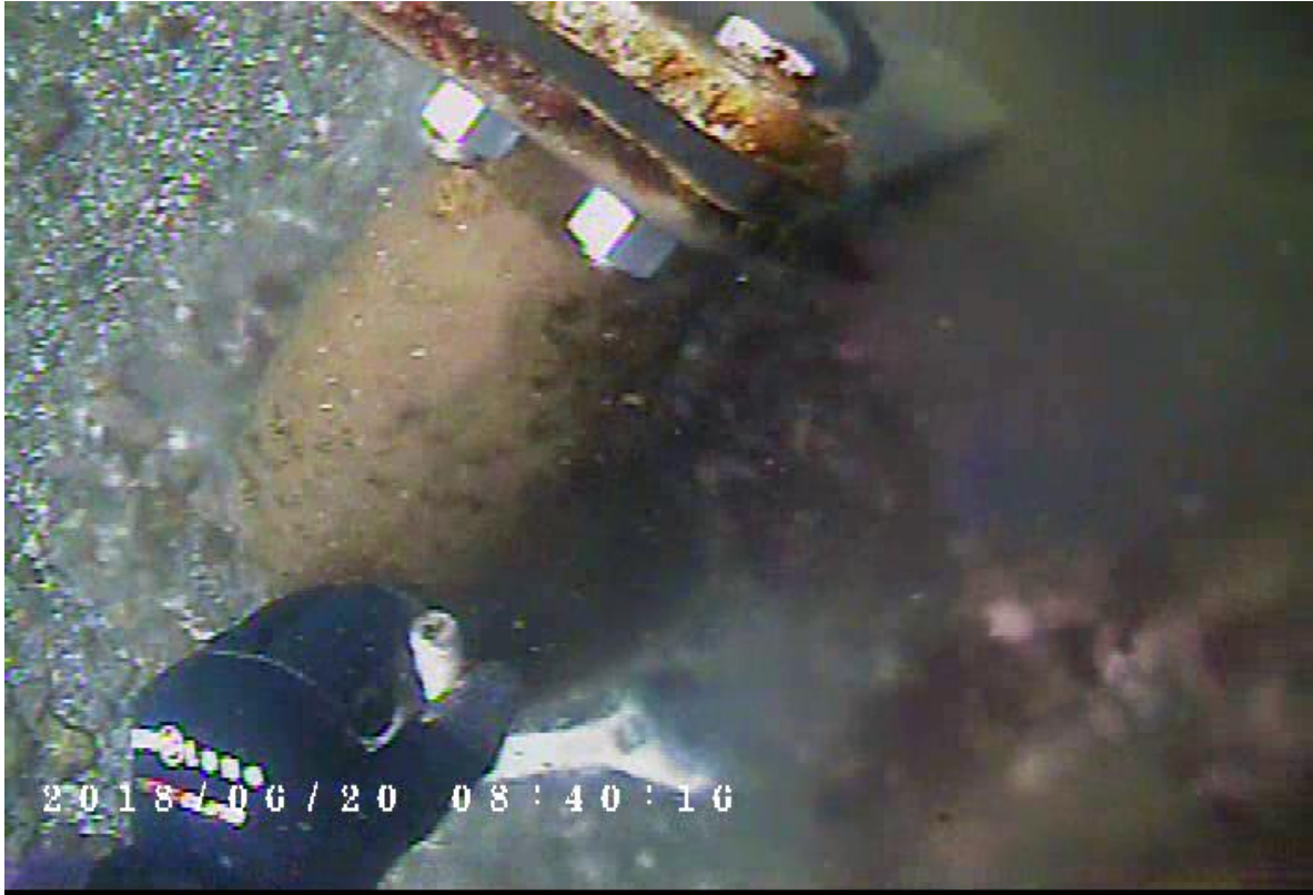
Photo 1 – Diffuser 1 showing strong flow
