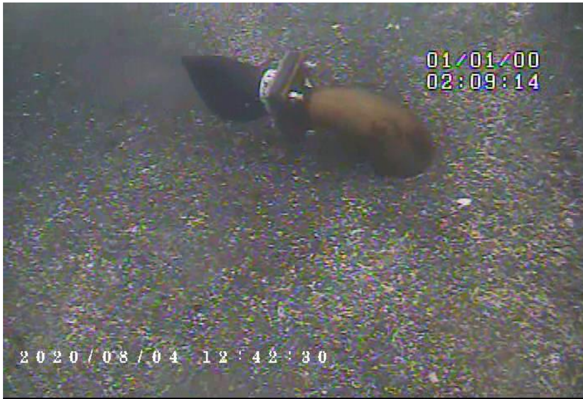
Photo 8 – Diffuser 8 showing strong flow
