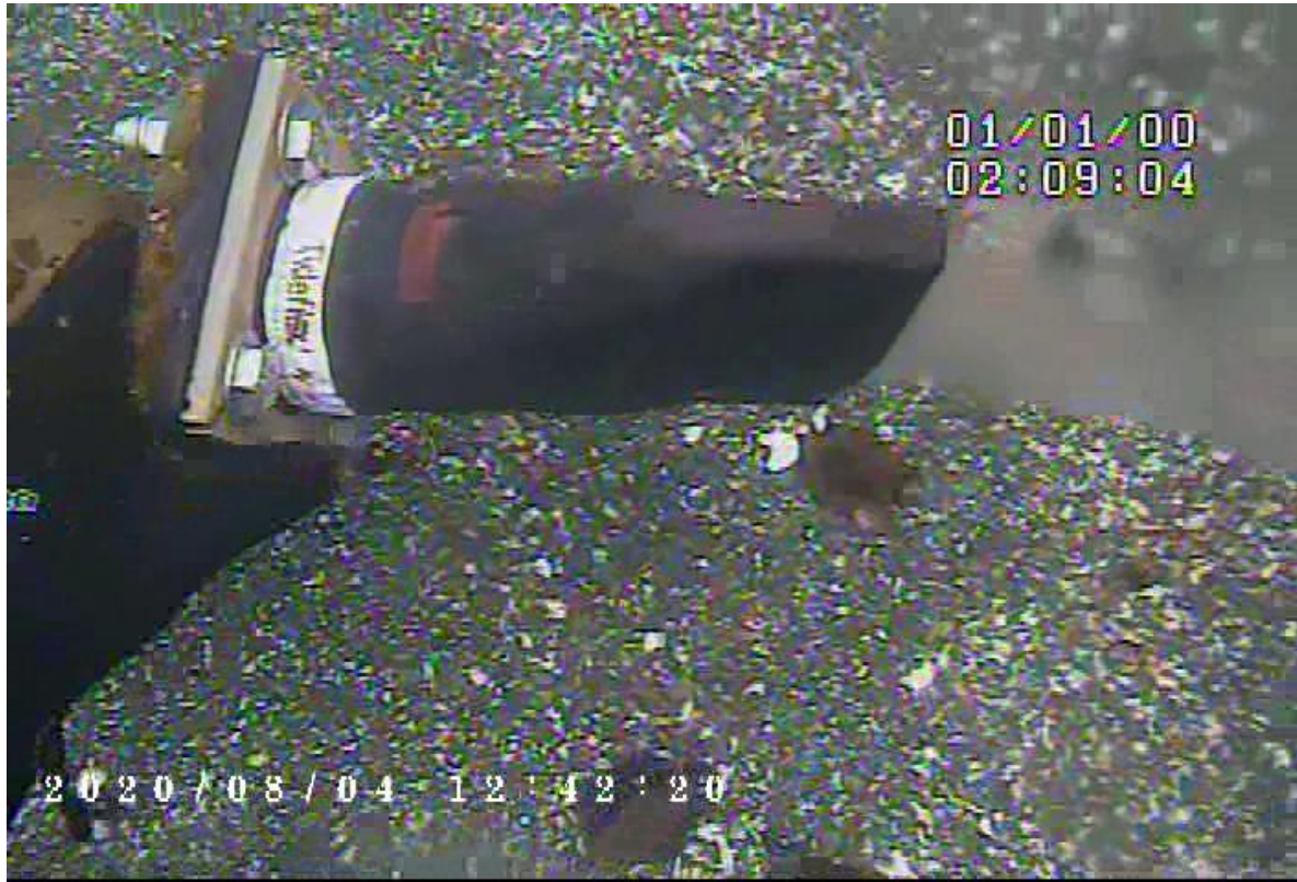
Photo 7 – Diffuser 9 showing strong flow
