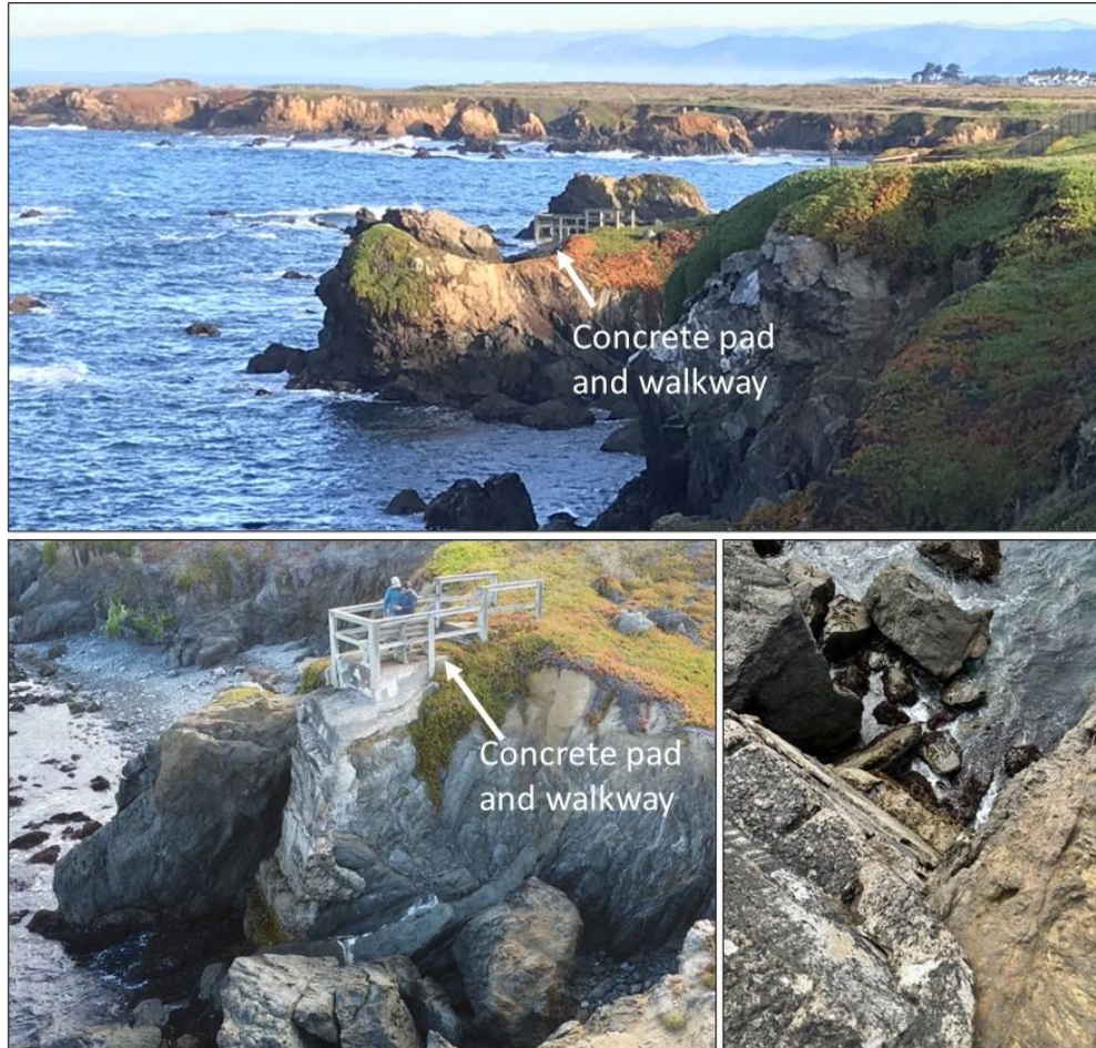
Figure 6. Concrete pad and walkway at top of rocky outcrop to which permeate pipeline may be attached.
