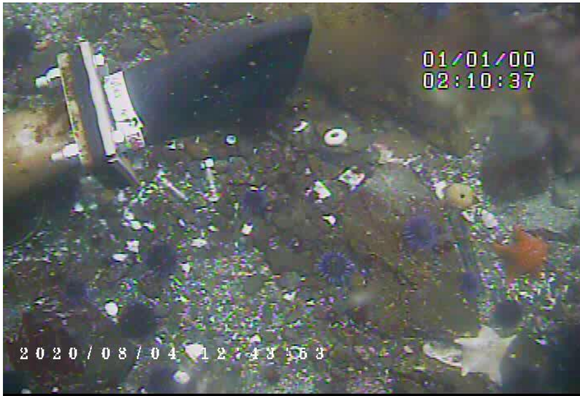
Photo 13 – Diffuser 3 showing strong flow
