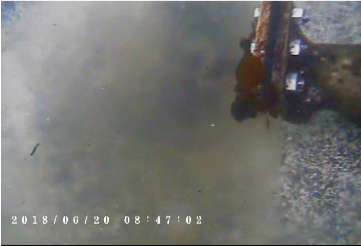
Photo 9 – Diffuser 9 showing strong flow
