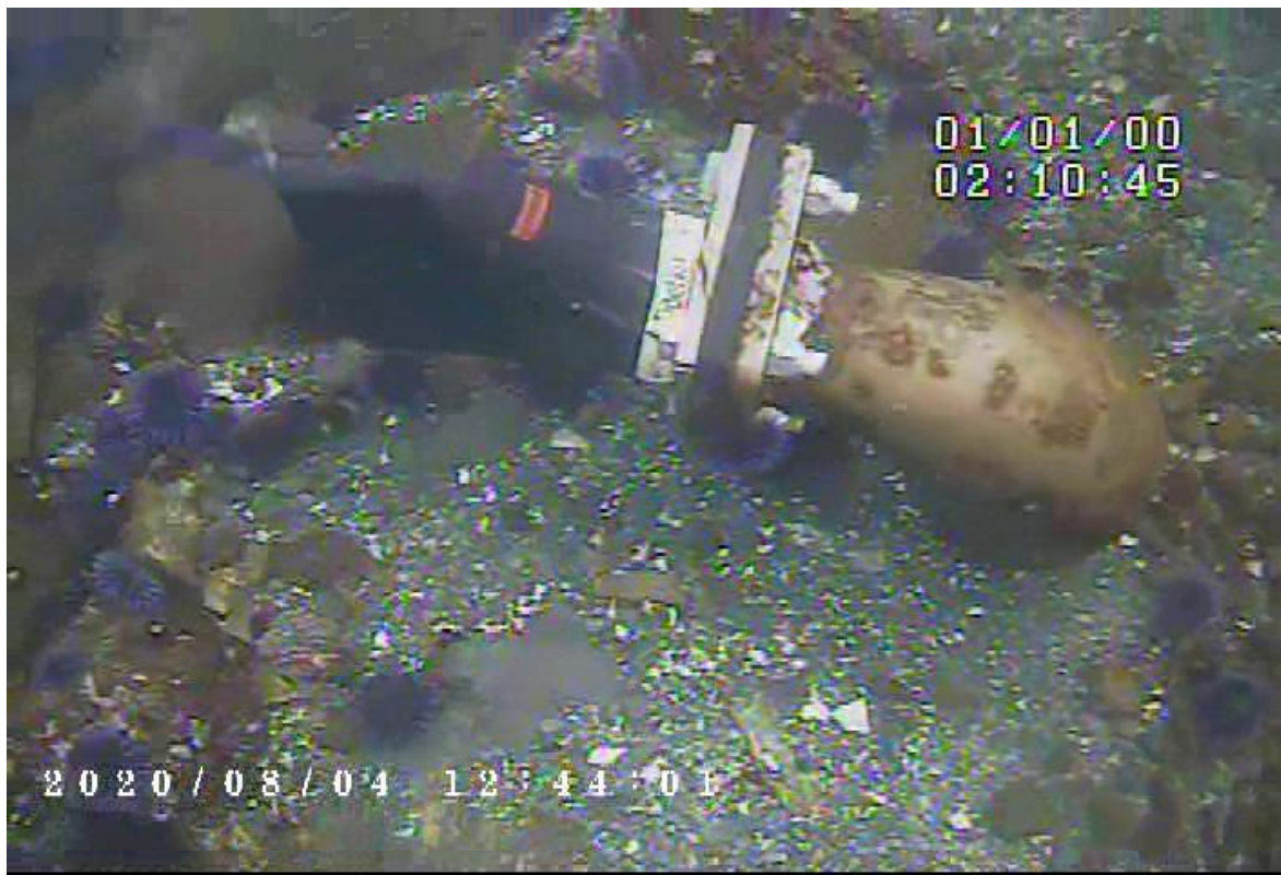
Photo 14 – Diffuser 2 showing strong flow
