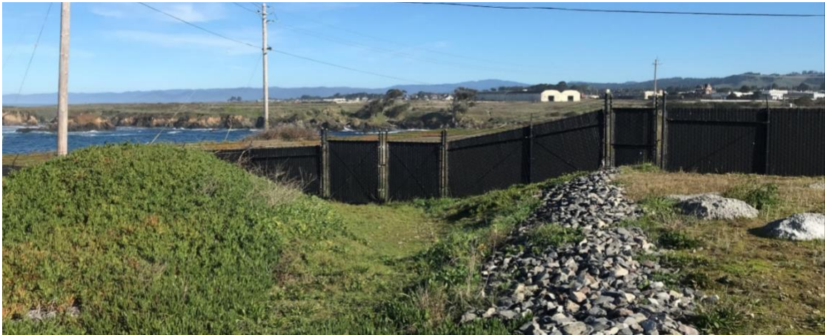
Figure 3. Fencing surrounding the Fort Bragg Wastewater Treatment Plant
