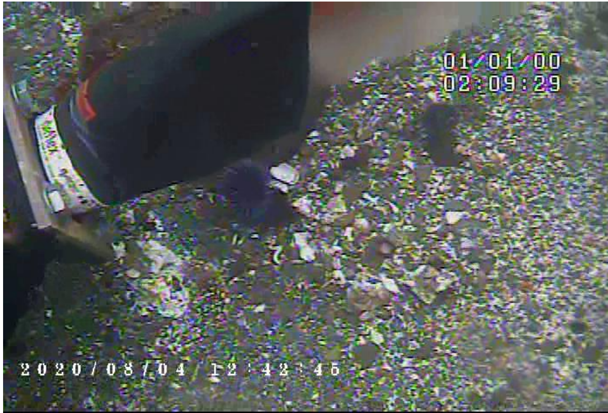
Photo 9 – Diffuser 7 showing strong flow
