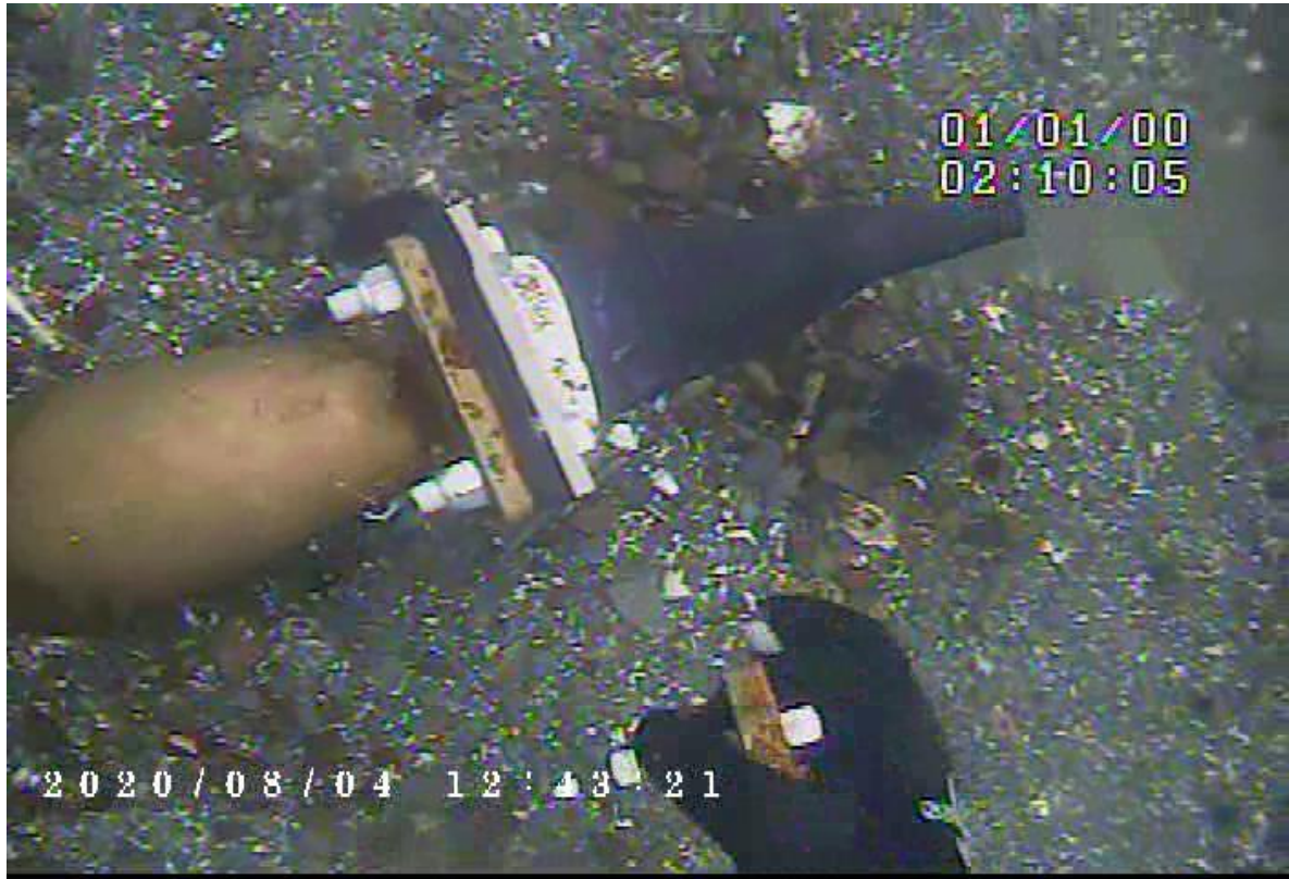
Photo 11 – Diffuser 5 showing strong flow
