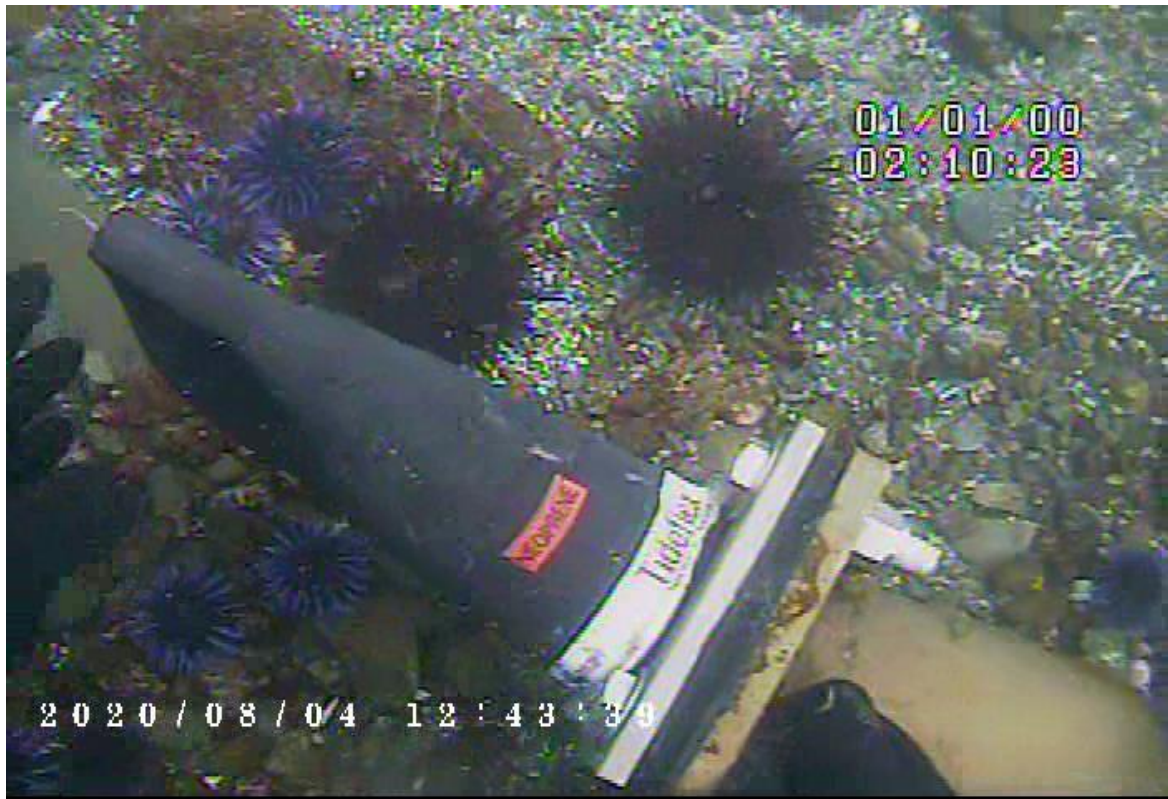
Photo 12 – Diffuser 4 showing strong flow
