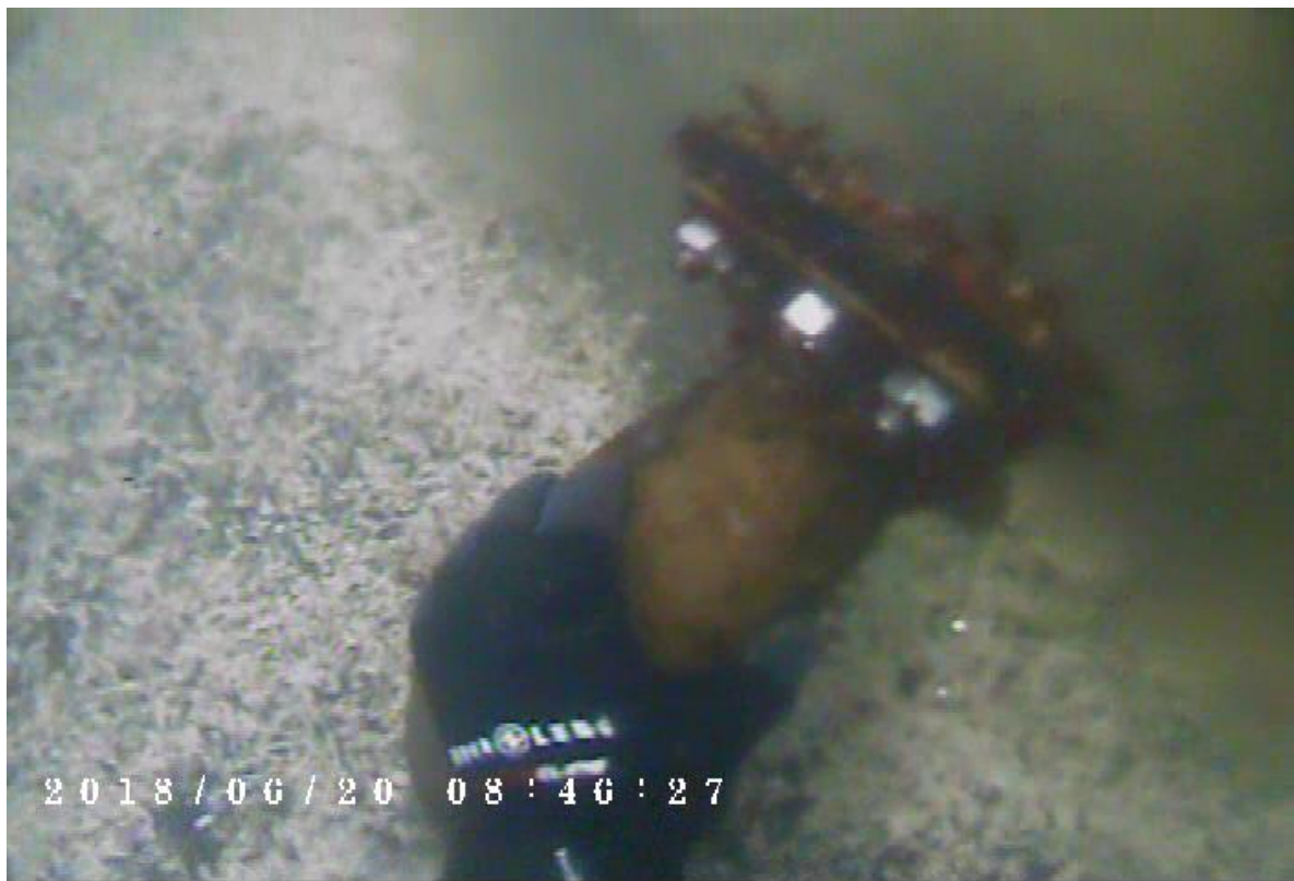
Photo 8 – Diffuser 8 showing strong flow
