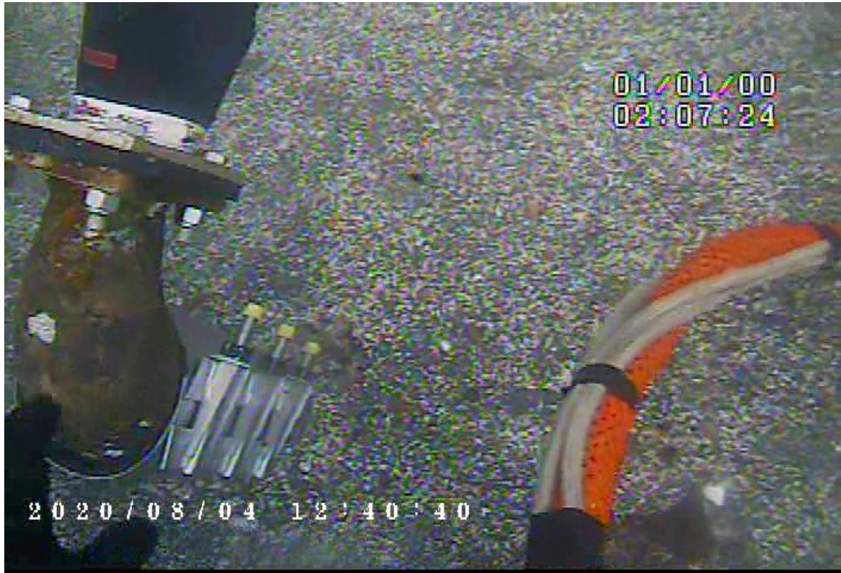
Photo 1 – Diffuser 14 clamp repair
