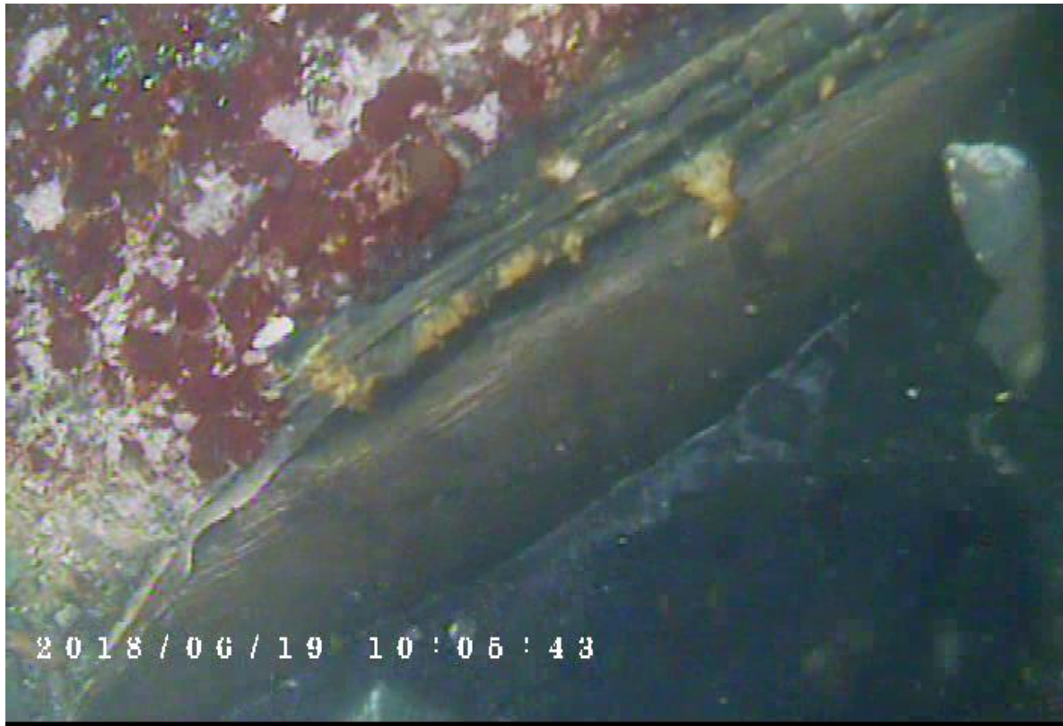
Photo 15 – Plywood bulkhead at the end of concrete encasement
